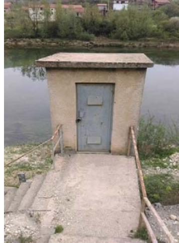
Slika 5. Automatska stanica Gorica prag Figure 5. Automatic station Gorica prag
